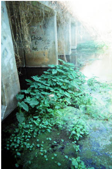
Vegetation at culvert #4 (west) inlet
