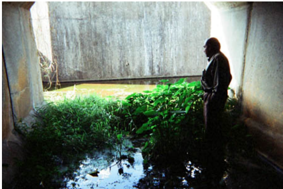
Vegetation at culvert #1 (east) inlet
