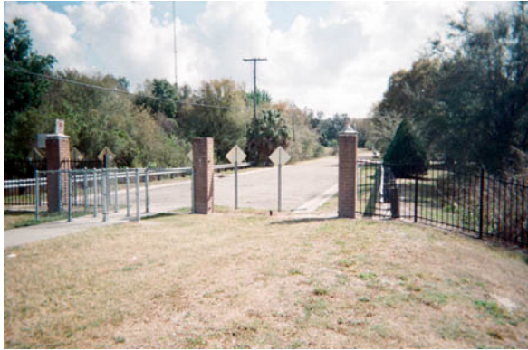
Missing fence on east side of dam
